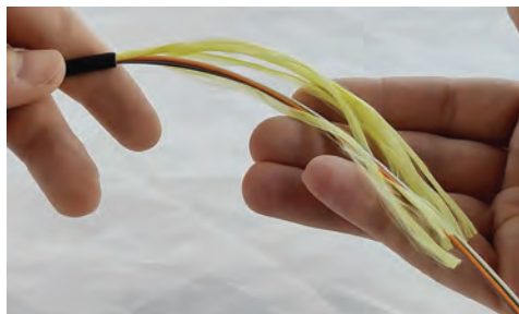
5. Trim Kevlar down to approximately 6-inches.
