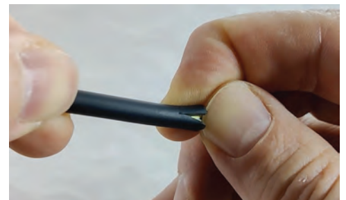
6. Slit the jacket approximately 1/4-inch on four sides.
